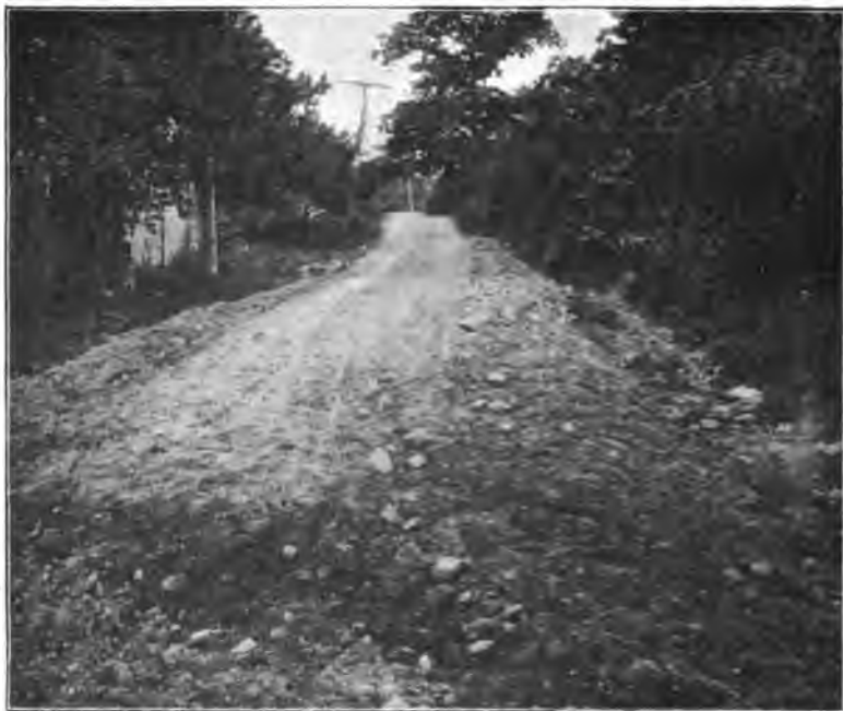
Sussex and Newton turnpike, Morris Co., before improvement.
